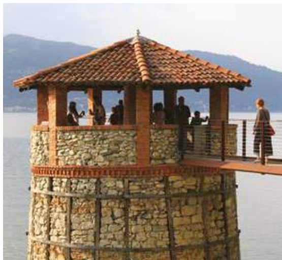
Lime kilns located at Lake Maggiore, Ispra, Italy. Since ancient times, lime has been the source for the manufacture of building materials, disinfectant and fertiliser. Sources: Peter Bosssew (left) and Tore Tollefsen (right).
