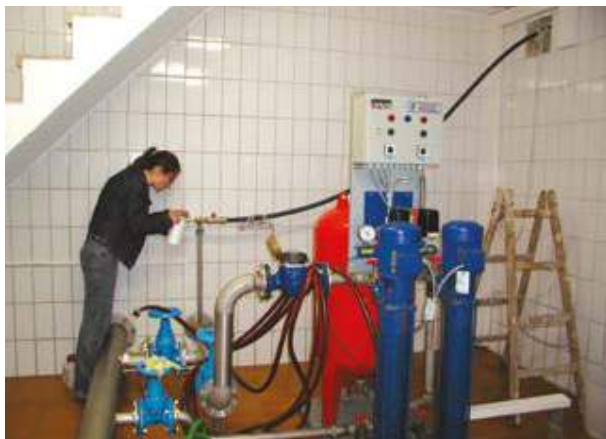
Water sampling in a pump house of a waterworks, Austria. Source: Valeria Gruber.
